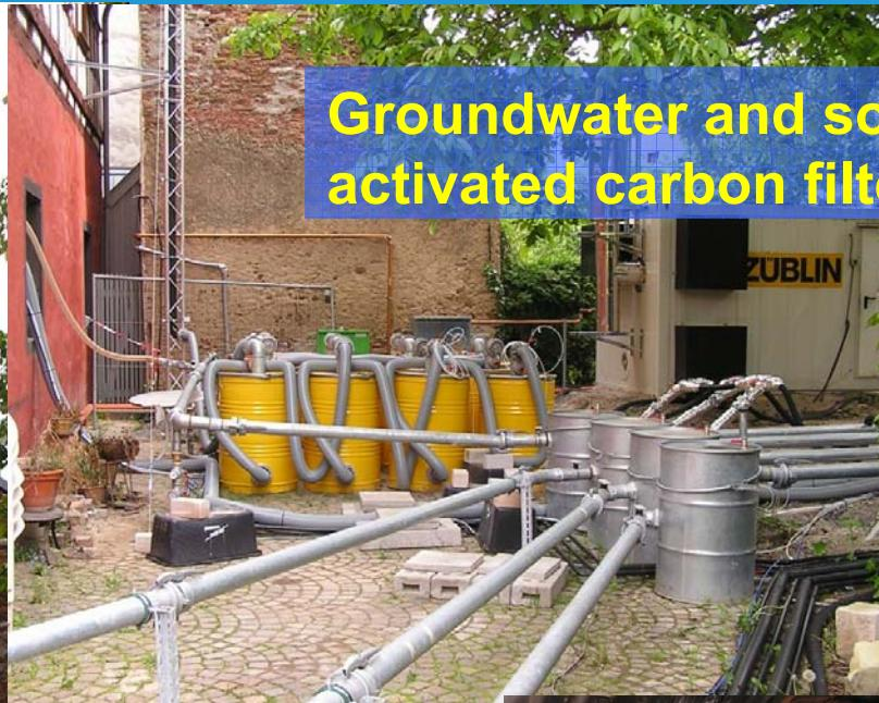
**Groundwater and soil vapour extraction,
